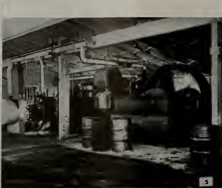
Fig. 4—Sandblasting is used on many operations in building tuna boats. Here, it is used for cleaning part of an ammonia coil for refrigerating system.
